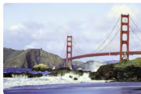
Golden Gate Bridge
